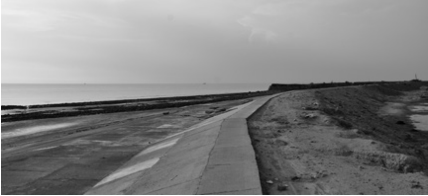
Fig 6.2. Seawall, Lighthouse, Sagar Island. Photo by author.
