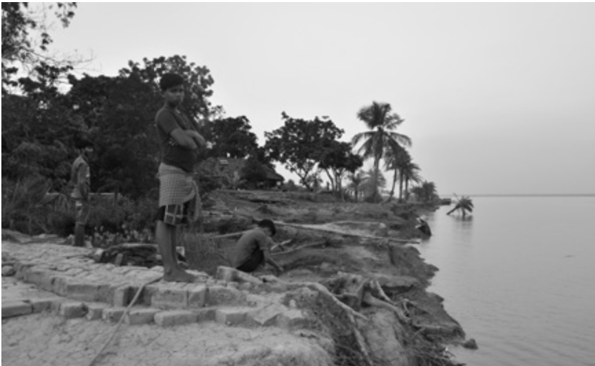
Fig 3.2. Erosion on high-land shores, Ghoramara Island. Photo by author.
